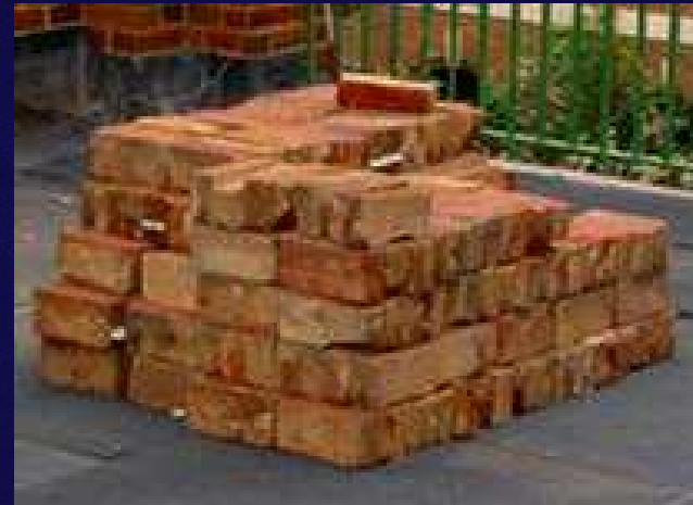
Removed brick saved for tooth-in and infill
